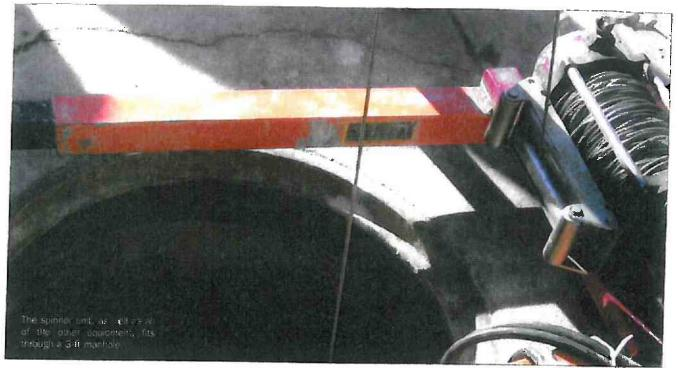
The underground gear that all fit through the 3-ft ID manhole openings included the Shotline spraying setup, nozzle, sled, winch and unique spinning head mounted on the sled. A five-man crew handled the process from mixing to final application. The winch speed was set based on the ID of the pipe, the overall desired thickness and the material volume pumped per minute.
